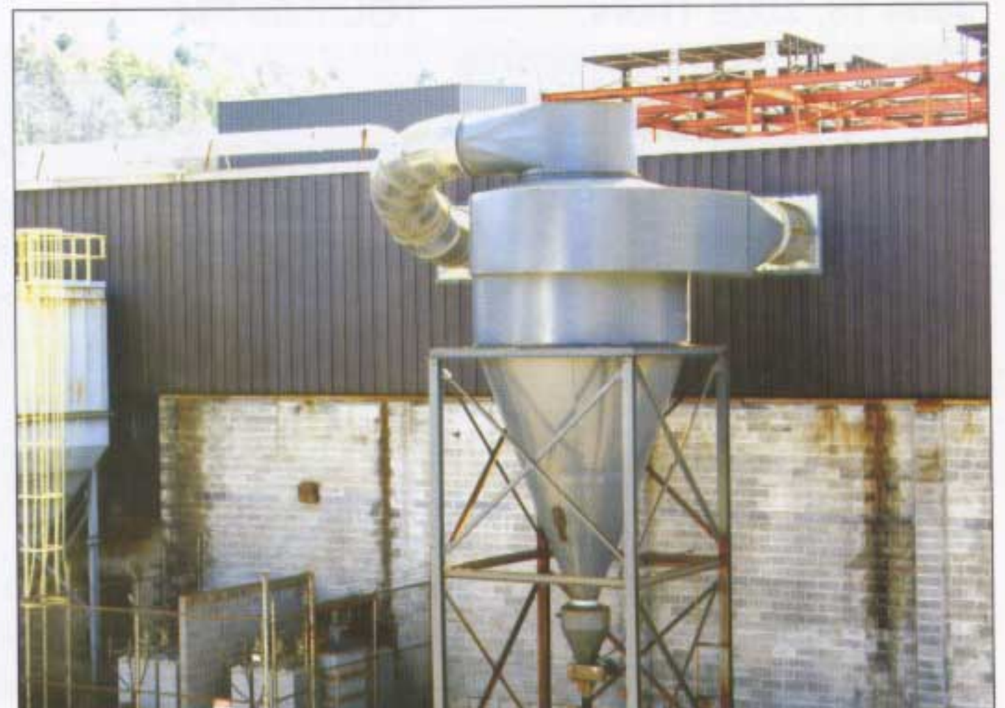
Cyclone upgrade to grinding room air handling system.
