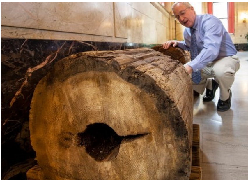
JT Hand, COO with the York Water Company, talks about the 1816 wooden water main recently extracted during a water main replacement project around Continental Square. The piece is on display in the lobby of the York Water Co. on East Market Street. (Photo: Paul Kuehnle, York Daily Record)
