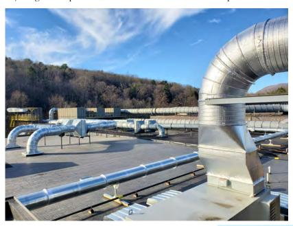
warm air is directed outside. During the winter months, the system recirculates the tempered, clean air back into the facility through pre-filters and
